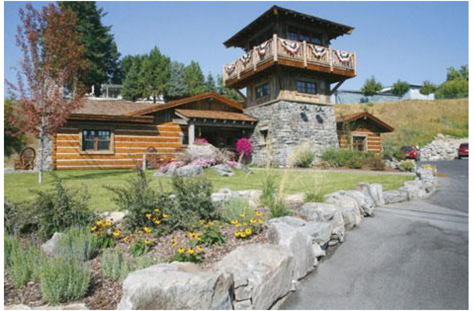
George Gibson designed the new Saddlehorn building on Grand Drive, and the finished product is catching everyone's eye. Mike Richeson - Bigfork Eagle
